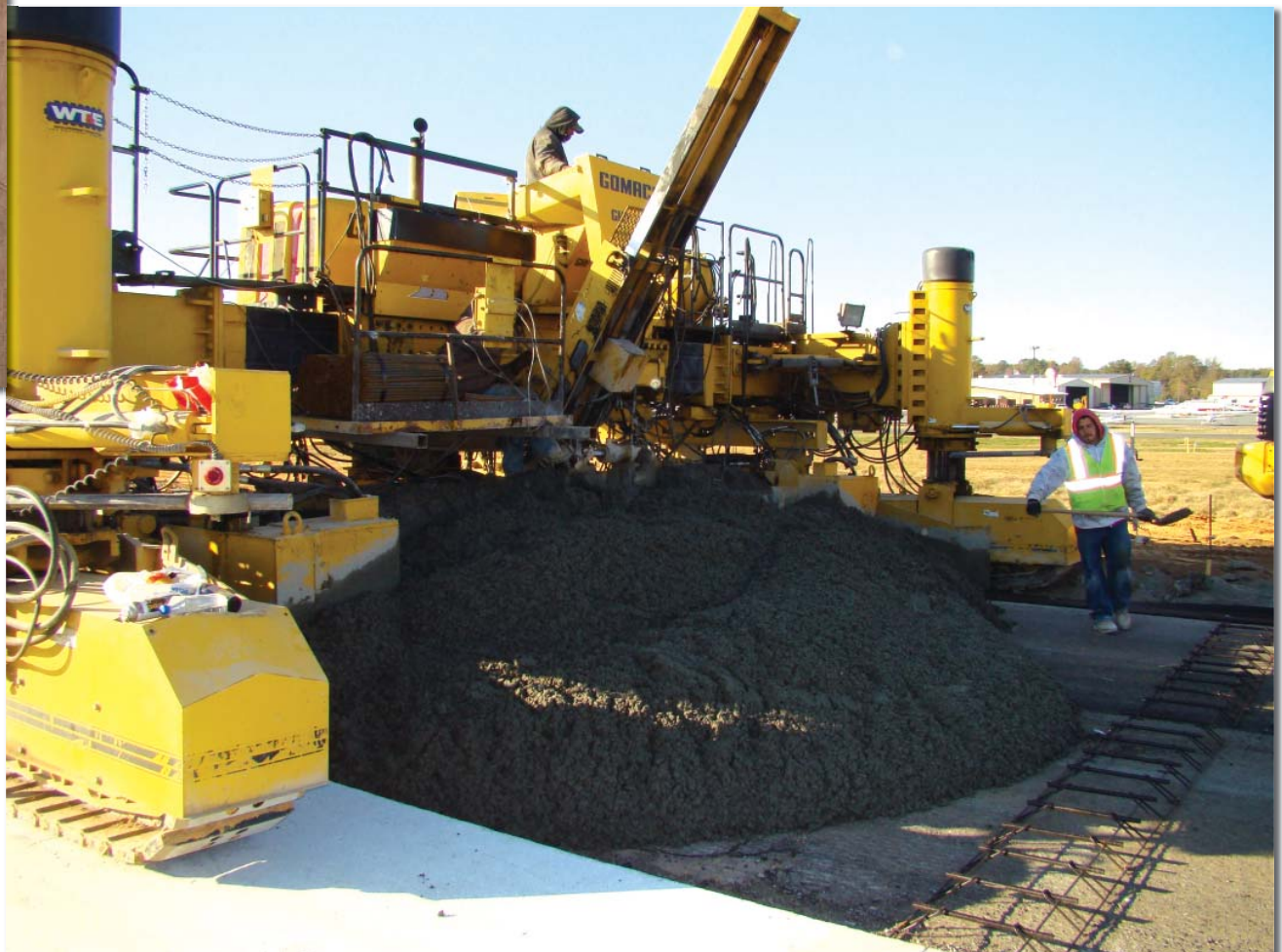
Above and below: A GOMACO 2800 paver placed concrete during the McCollum Airport runway rehabilitation project at a rate of 1,800 cubic yards of concrete per day.
