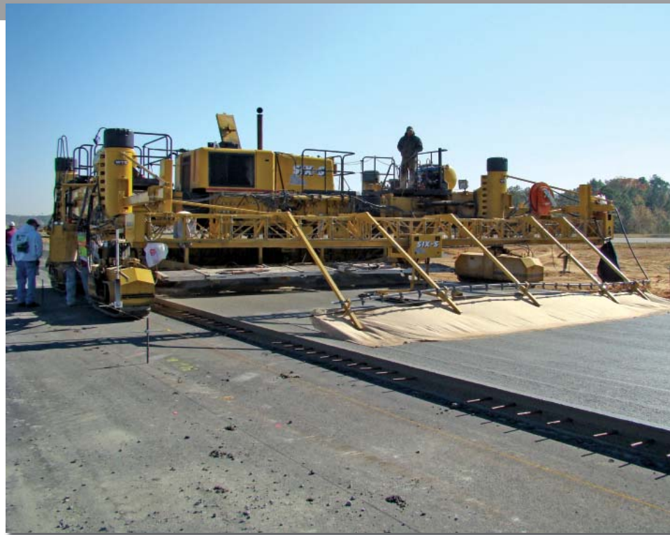
Above and below: A GOMACO 2800 paver placed concrete during the McCollum Airport runway rehabilitation project at a rate of 1,800 cubic yards of concrete per day.
