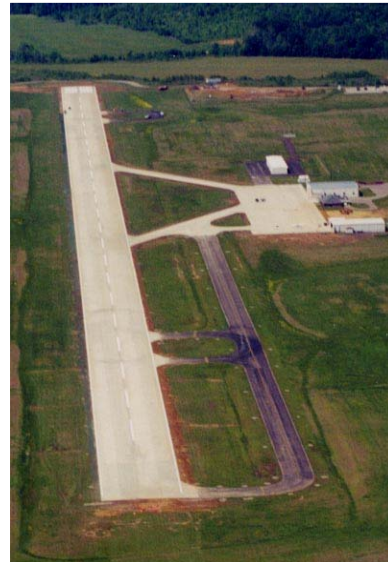
Photo 1: Savannah-Harding County Airport Whitetopping from the air.
