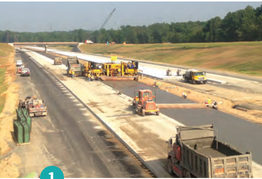
1 Paving underway on I-485
