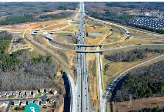
3 I-85/I-485 turbine interchange
