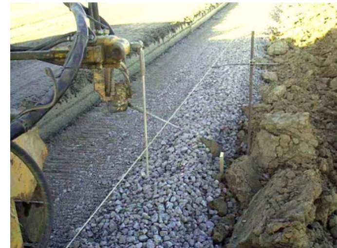
Stringline and paving hub alignment (from Minnesota DOT)
