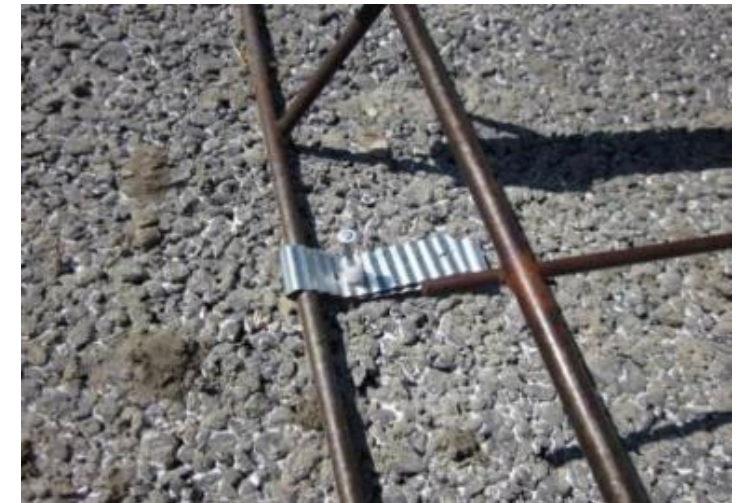
Dowel basket anchored to subgrade (upper) and existing asphalt (lower, b
