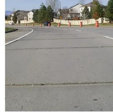
Faulted Joints
