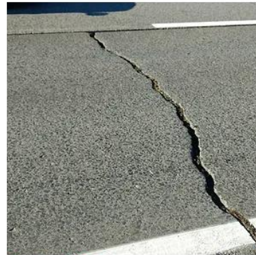
Cracked Slabs
