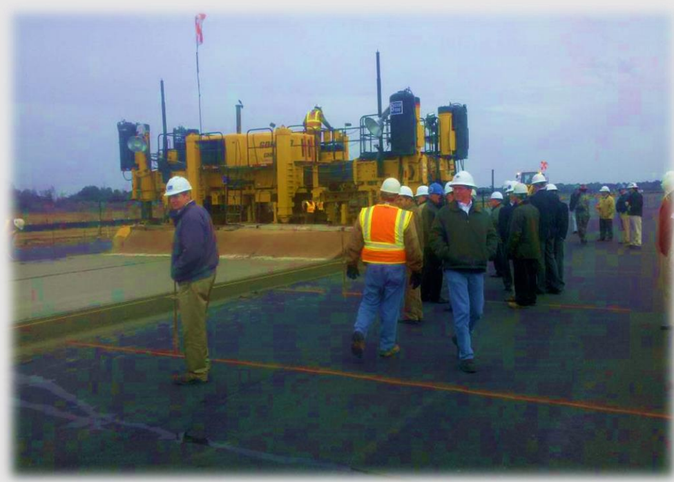
Charleston Exec Airport Concrete Overlay of Concrete
