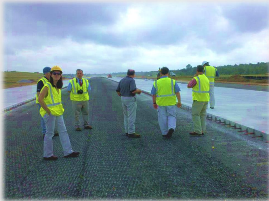
Lancaster County Airport Concrete Overlay of Asphalt
