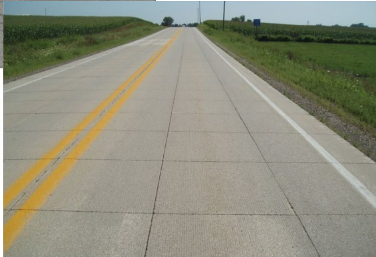
SH-13 Bonded Overlay 6'x6' Joint Spacing (2014)
